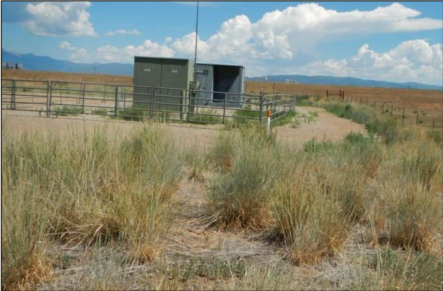
Photo 3. View the eastern project area from the southeastern corner facing northward.
