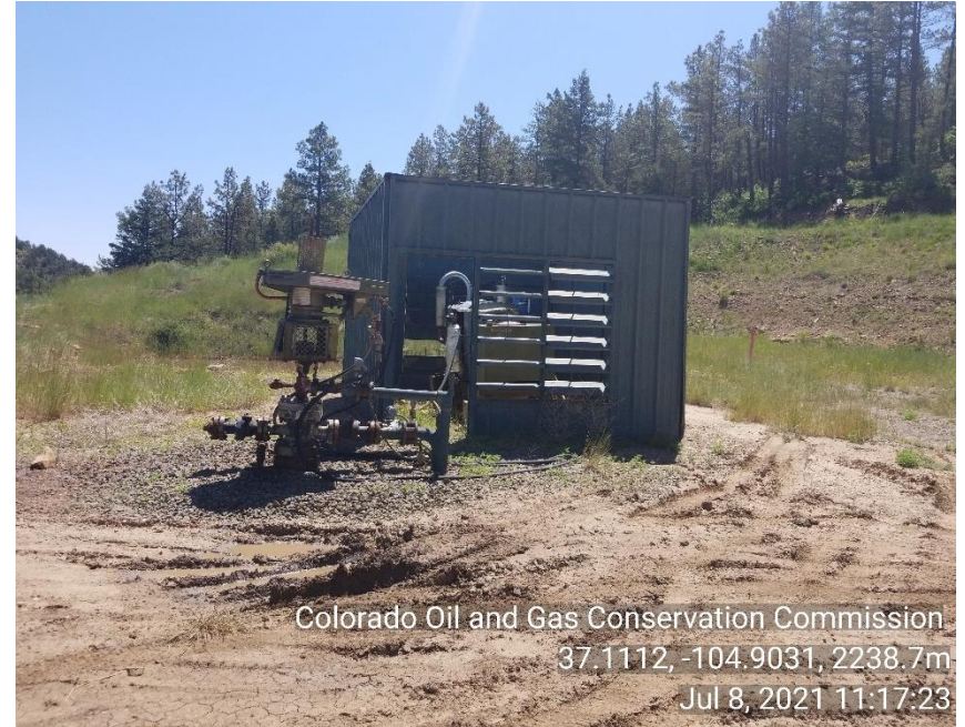
Photo 4 AC 5-09V Well head and motor skid
