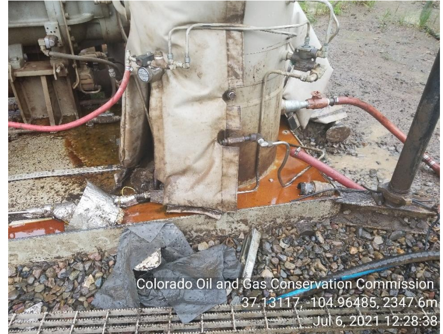
Photo 4 fluid in compressor skid about to run over.
