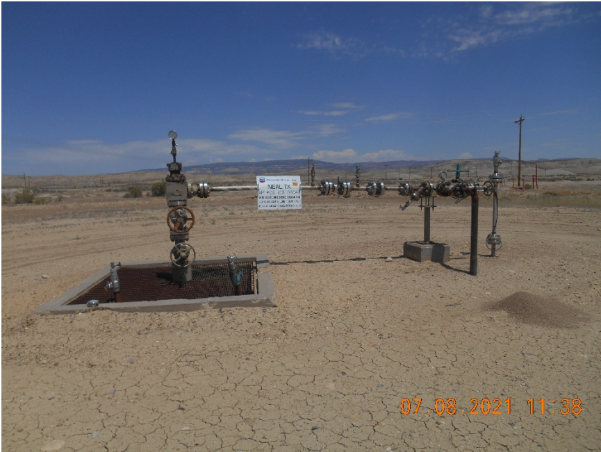
Injection wellhead
