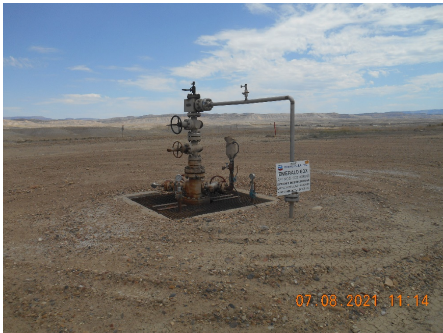
Injection wellhead
