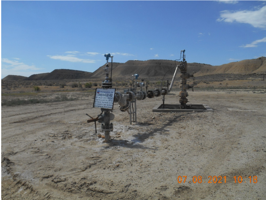
Injection wellhead. Water disposal well.
