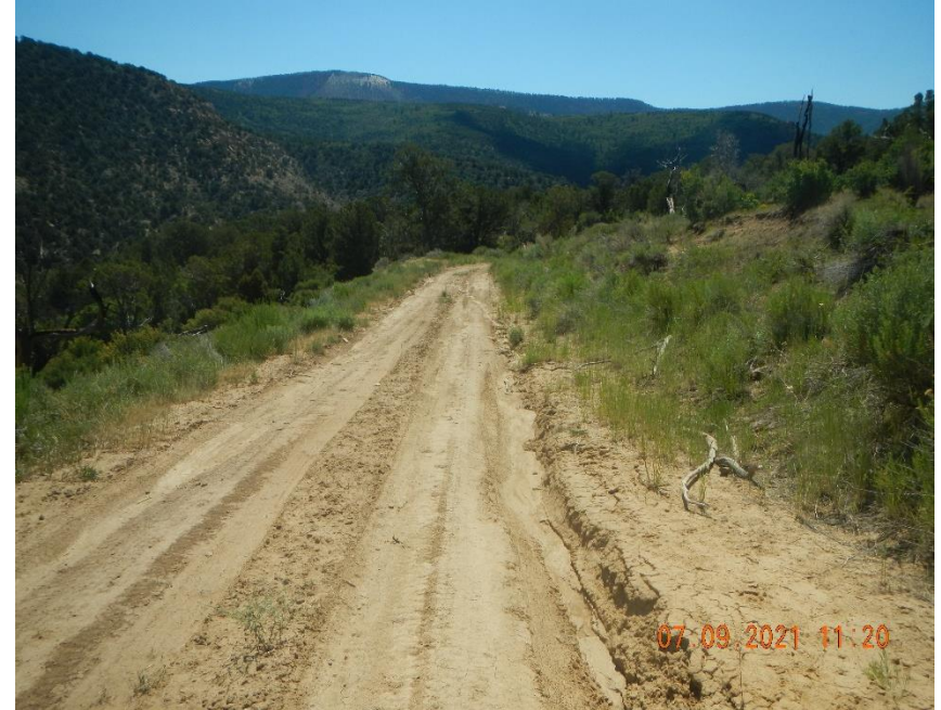
Access road and ditch need maintained.
