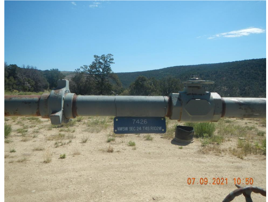
No api# on well tag/sign
