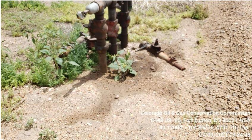
**Photo 3 stained soil by flow line manifold**
