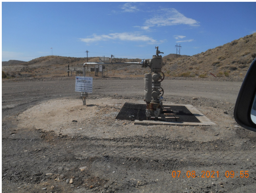
Injection wellhead
