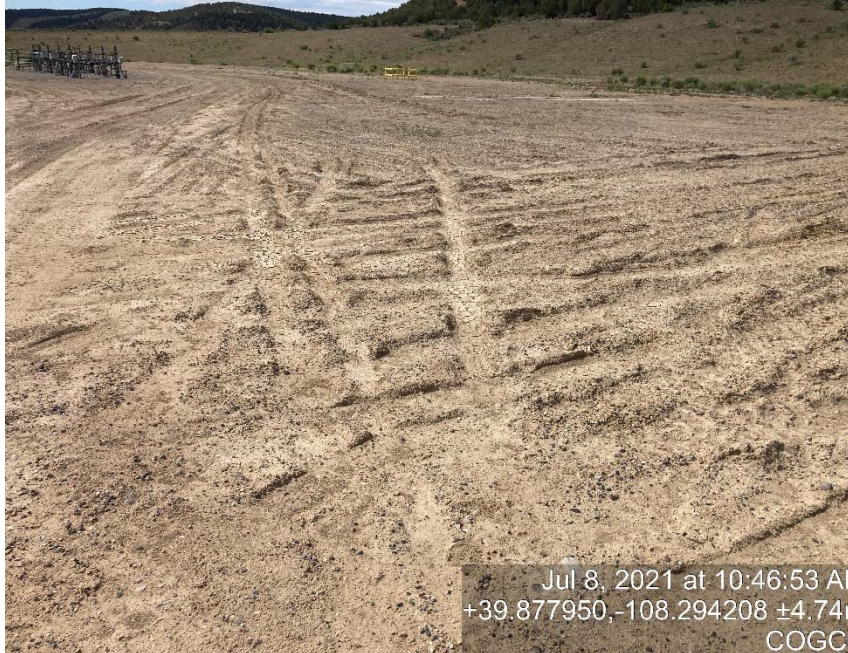
Lack of stabilization/compaction
