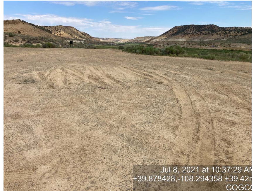
Lack of stabilization/compaction
