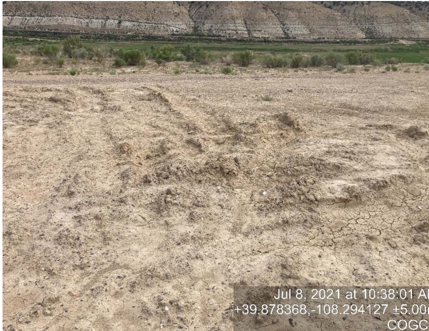
Lack of stabilization/compaction
