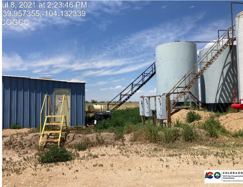
Pic 5 stored equipment/weeds/tanks
