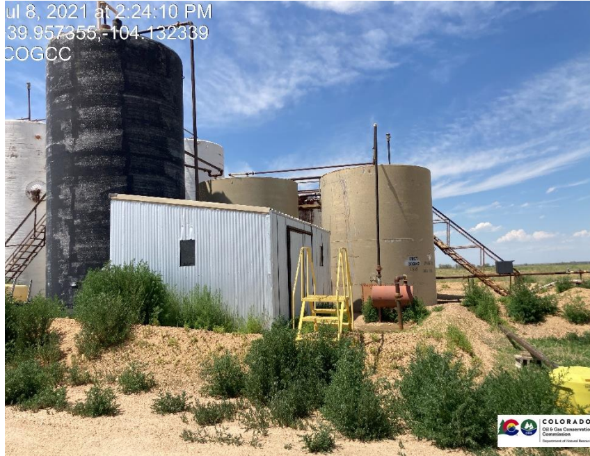
Pic 7 tanks, weeds.
