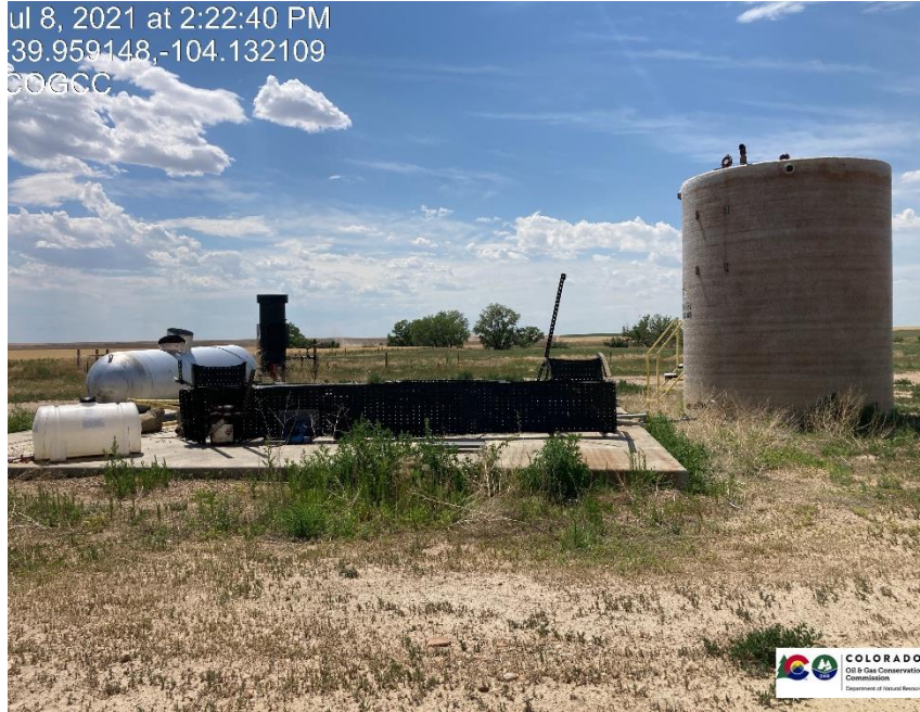
Pic 1 stored equipment
