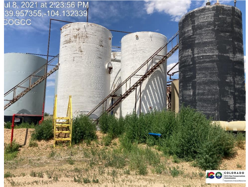
Pic 6 weeds, tanks
