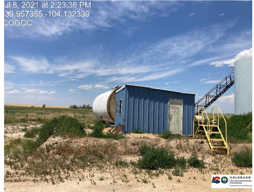
Pic 4 stored equipment
