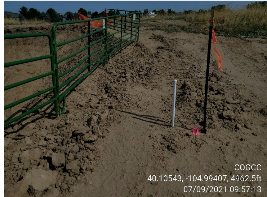
Photo 6 Piezometer located east of excavation
