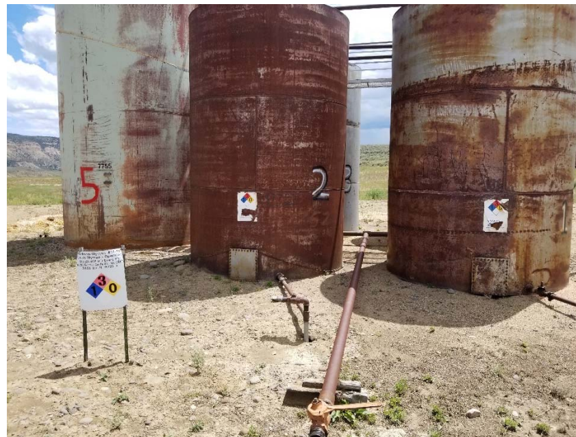
Photo 3. Tank labels incomplete.
