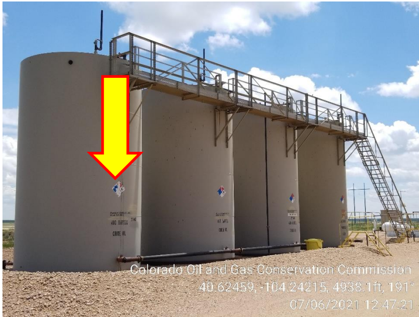
Photo 1 – Tank Battery, NFPA Label
