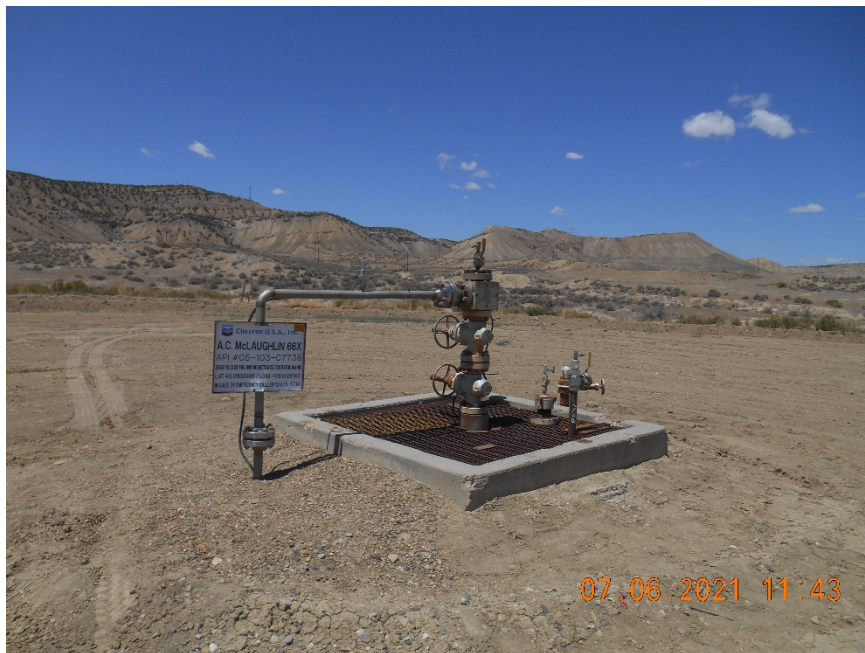
Injection wellhead
