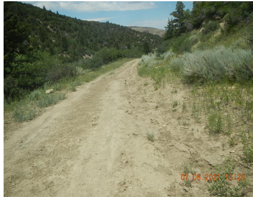
Road and road BMPs not maintained. From location Steele-B 7413 to location FOUNDATION CREEK B 7407
