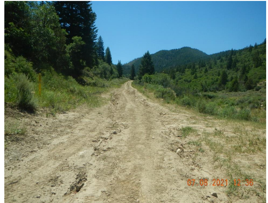
Road and road BMPs not maintained. From location Steele-B 7413 to location FOUNDATION CREEK B 7407
