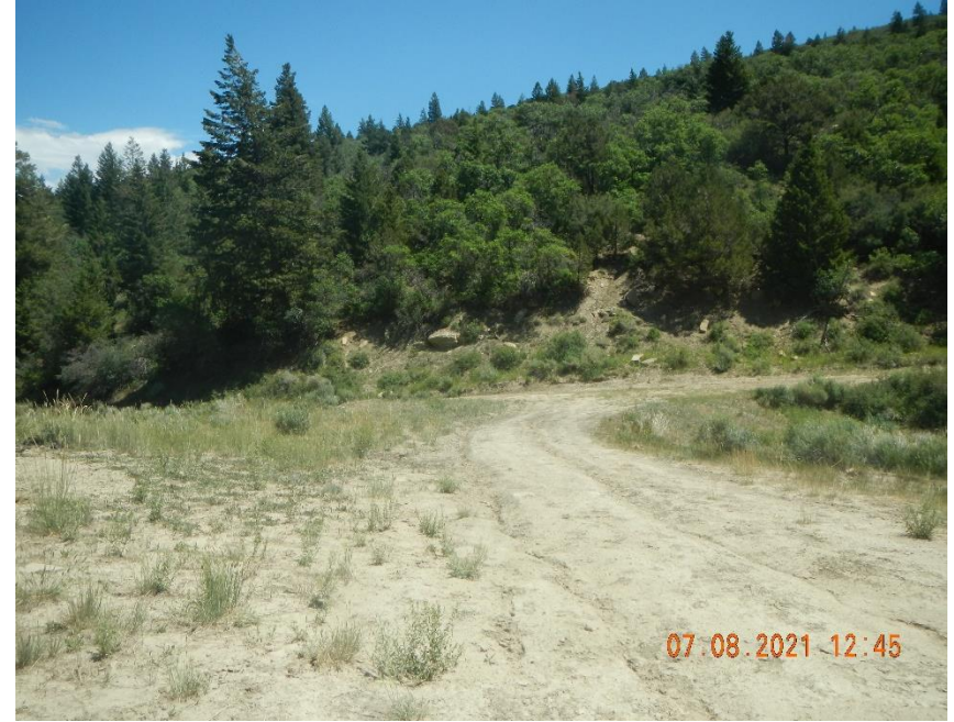
Ruts washing from location to access intersection.
