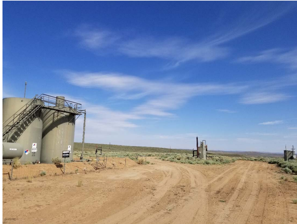
Photo 1. Overview of location taken facing north.
