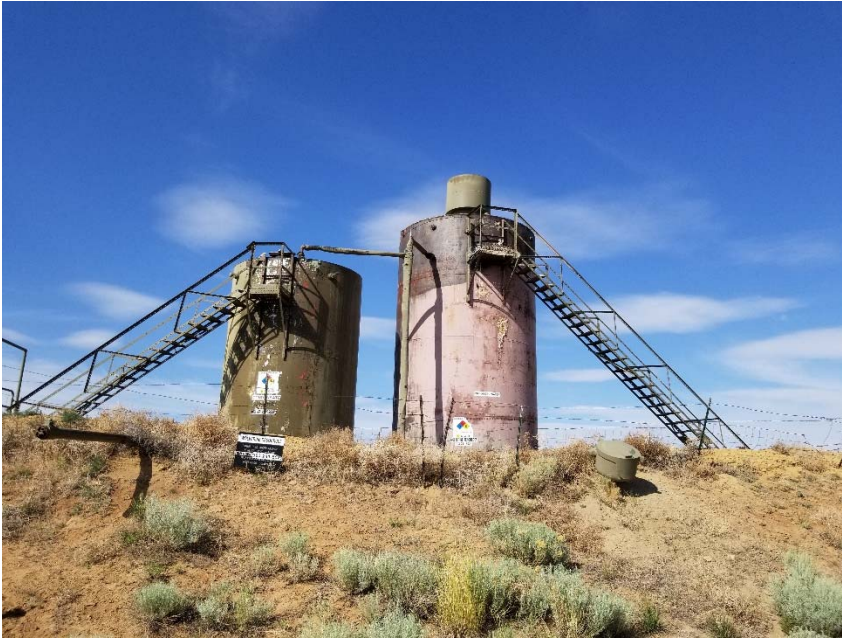
Photo 3. Incomplete tank labels. Annual weeds on location.
