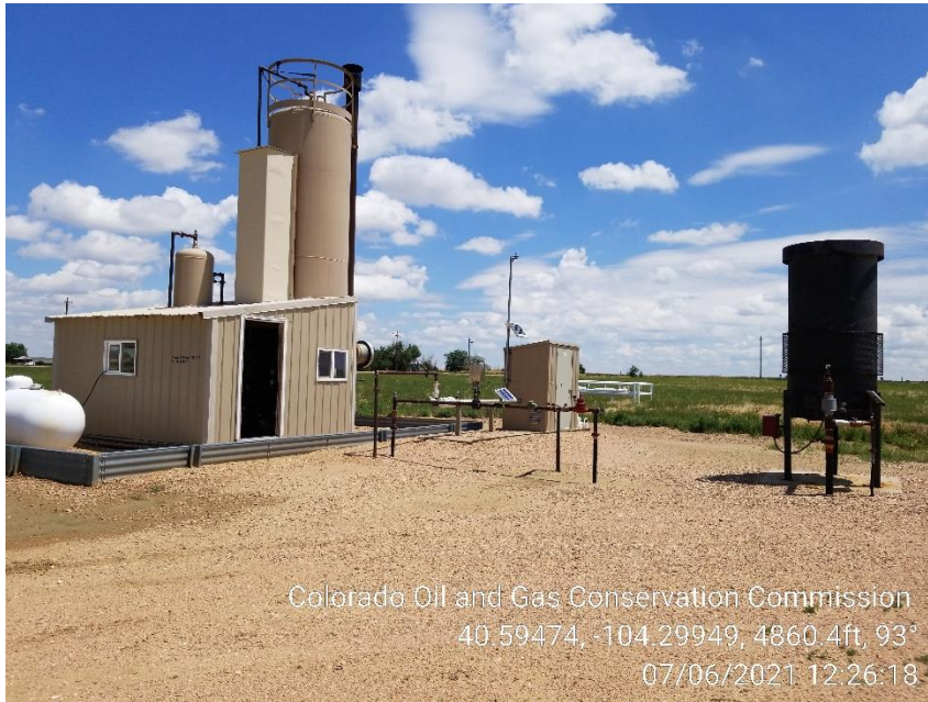
Photo 3 – Heater Treater, Gas Meter and ECD
