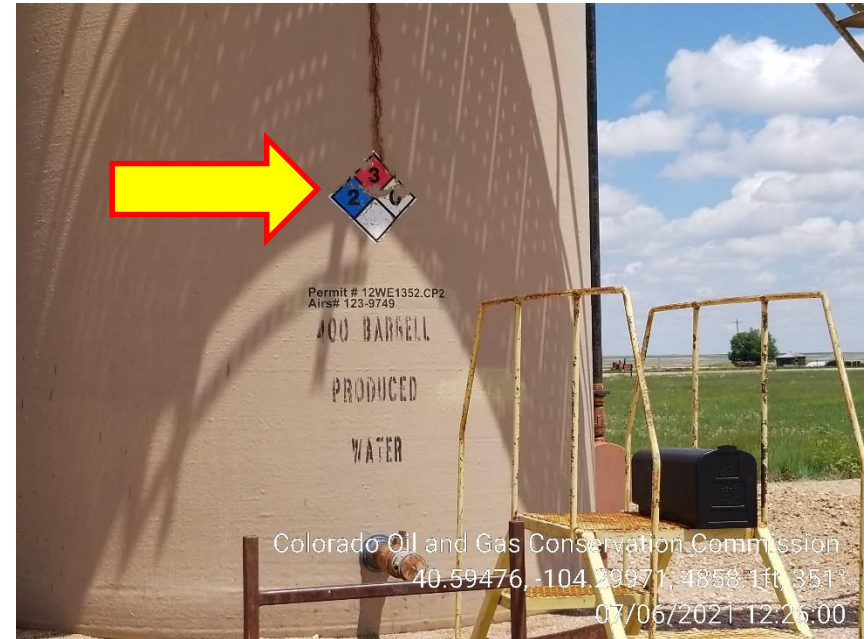
Photo 6 – NFPA Label is Fading
