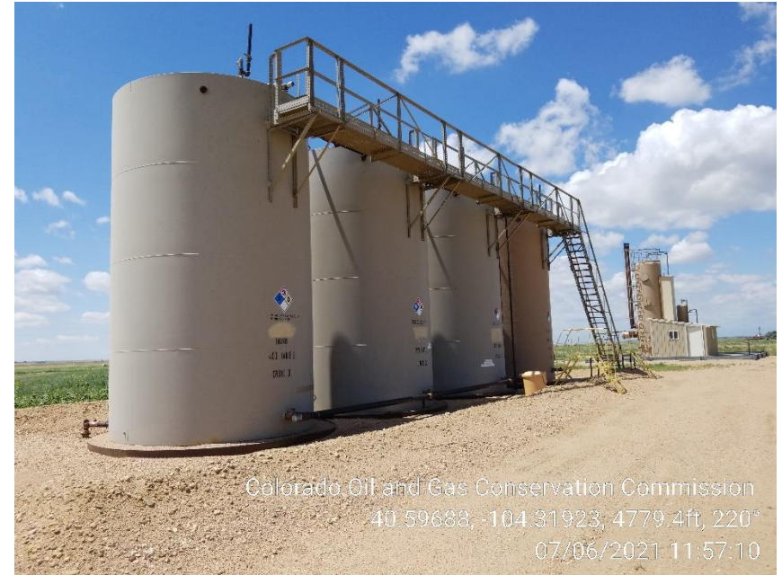
Photo 2 – Tank Battery
