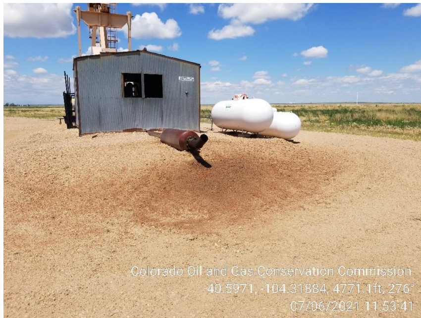
Photo 7 – Stained Soil at Exhaust
