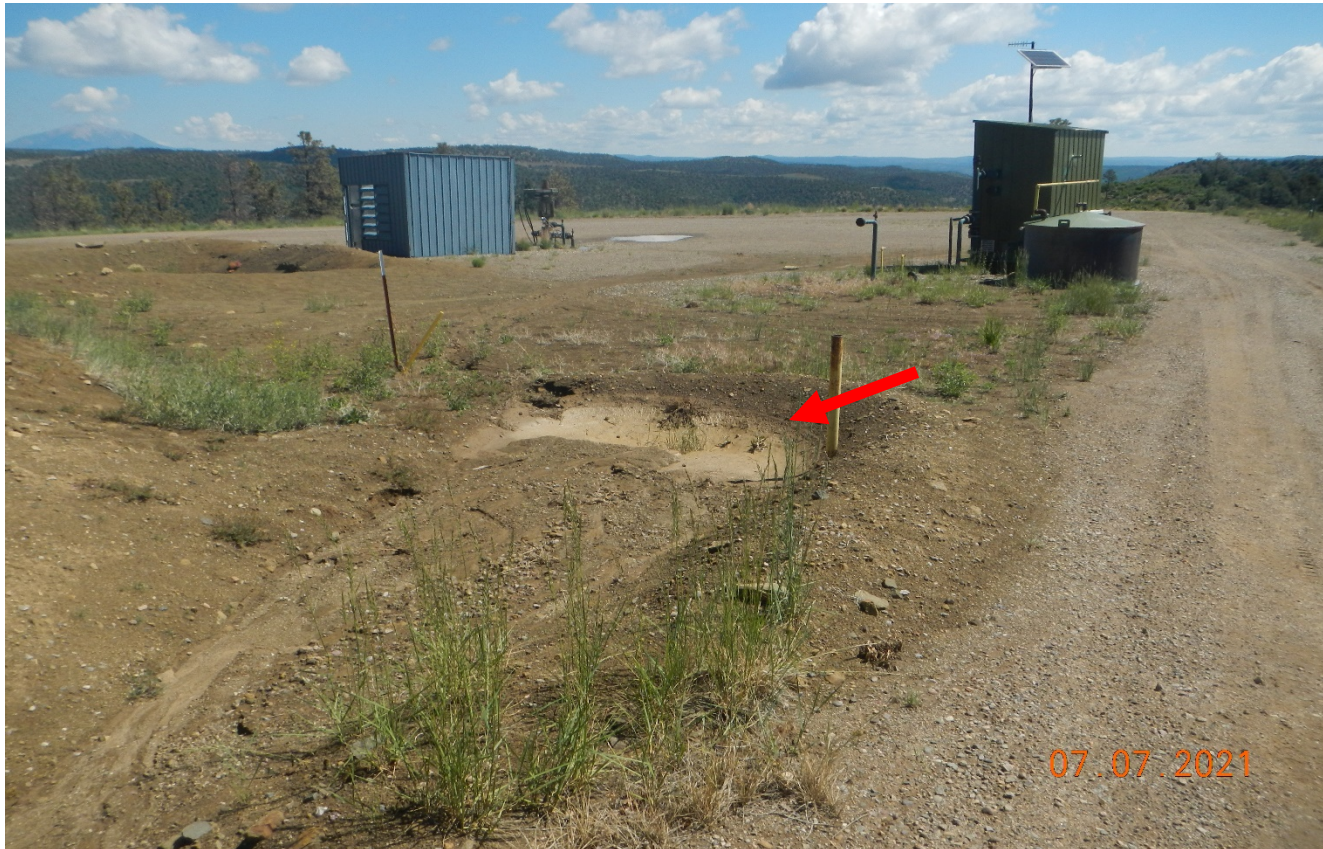
Photo 3. Facing northeast at the well site. The culvert shown at red arrow is filled in with sediment.
