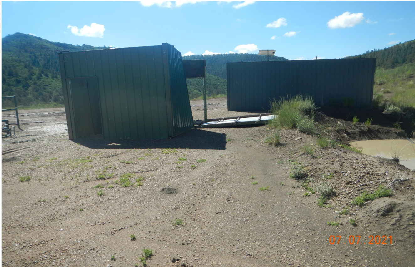
Photo 4. Facing toward the equipment. A panel is laying on the ground and needs to be re-installed.
