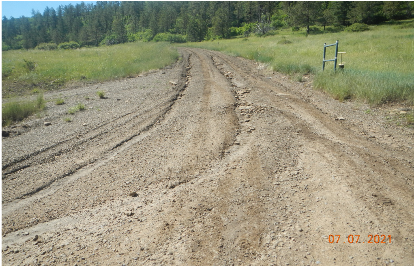
Photo 1. Facing southeast along the access road. The road is not stabilized and there are signs of erosion.
