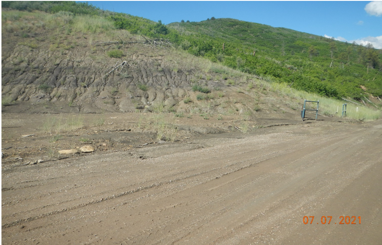
Photo 3. Facing southwest at the location. Erosion of the cut slope is directing sediment down towards the road. This area needs to be stabilized erosion controls are needed (e.g. sediment trap)
