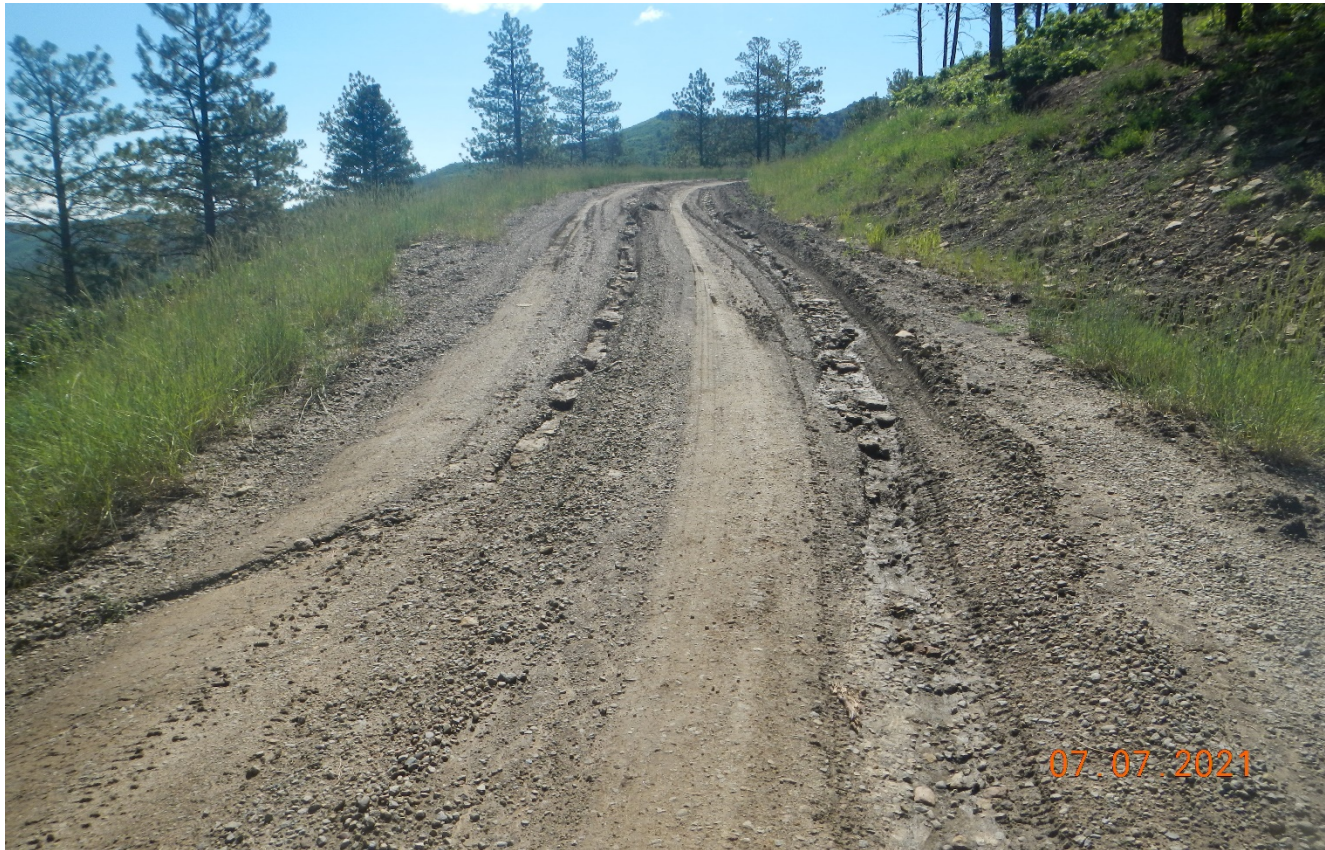
Photo 2. Facing southeast further along the access road. The road is not stabilized and there are signs of erosion and vehicle rutting.
