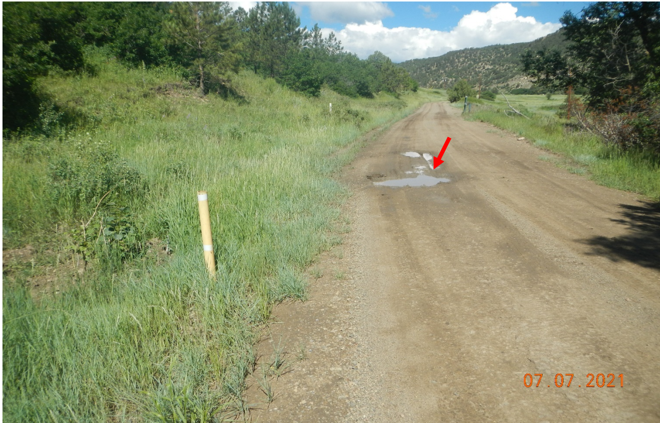
Photo 3. Additional grading will be needed to drain stormwater toward the culvert in this area. Stormwater is already accumulating on the road shown at red arrow. Lat/Long:37.06585,-104.93198.
