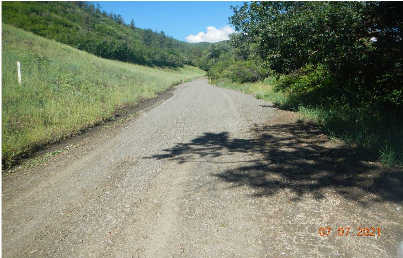
Photo 1. The road was regraded and gravel was applied to areas of the road.
