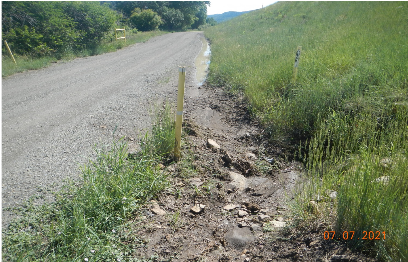
Photo 2. It appears recent rain events have deposited sediment into the culverts. Ongoing maintenance needs to be performed.
