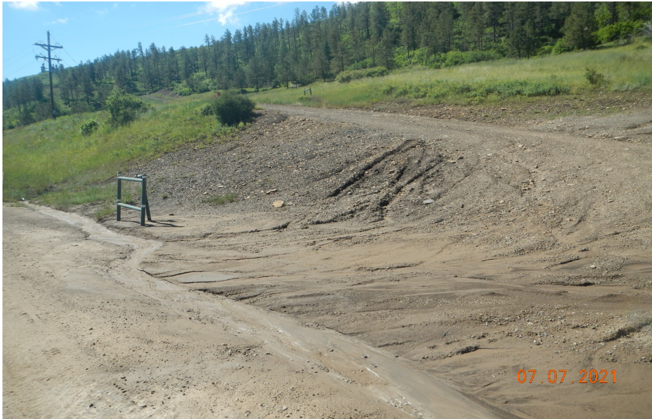
Photo 4. Facing southeast toward the access road. Stormwater is directed toward the culvert shown at red arrow. Sediment is already filling into this area which will require ongoing maintenance.
