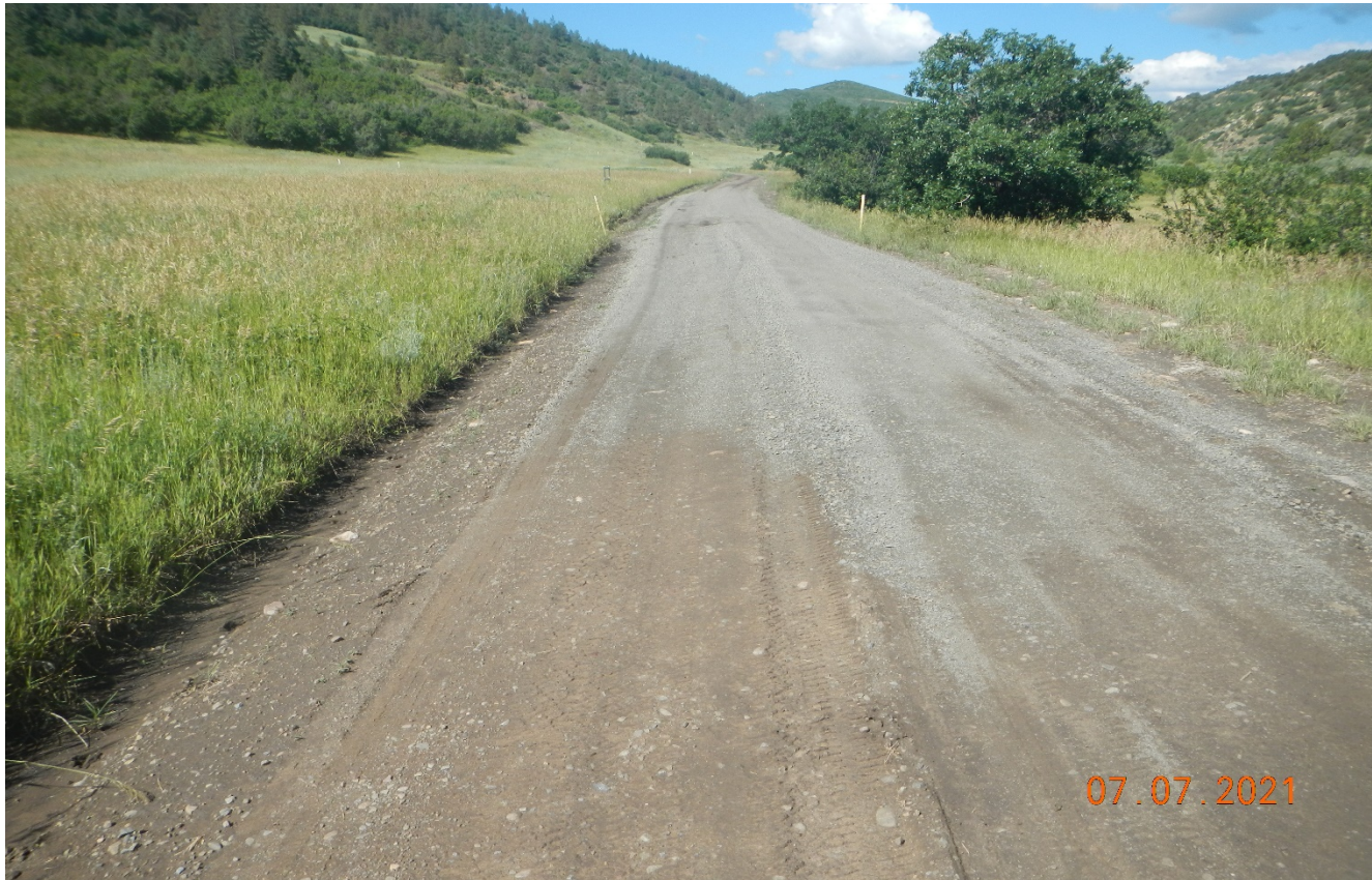
Photo 2. The road was regraded and gravel was applied to area of the road.
