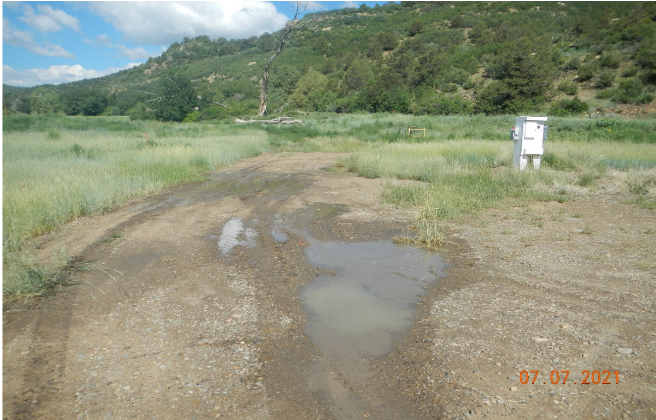
Photo 10. There does appear to be gravel toward the drip line. Additional gravel may be needed toward the drip line to prevent rutting.
