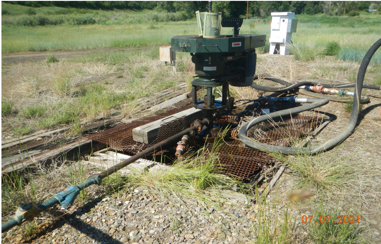
Photo 7. There is an opening where the steel grate is around the wellhead. This area needs to be covered to prevent wildlife entry. Previous corrective action was not performed.
