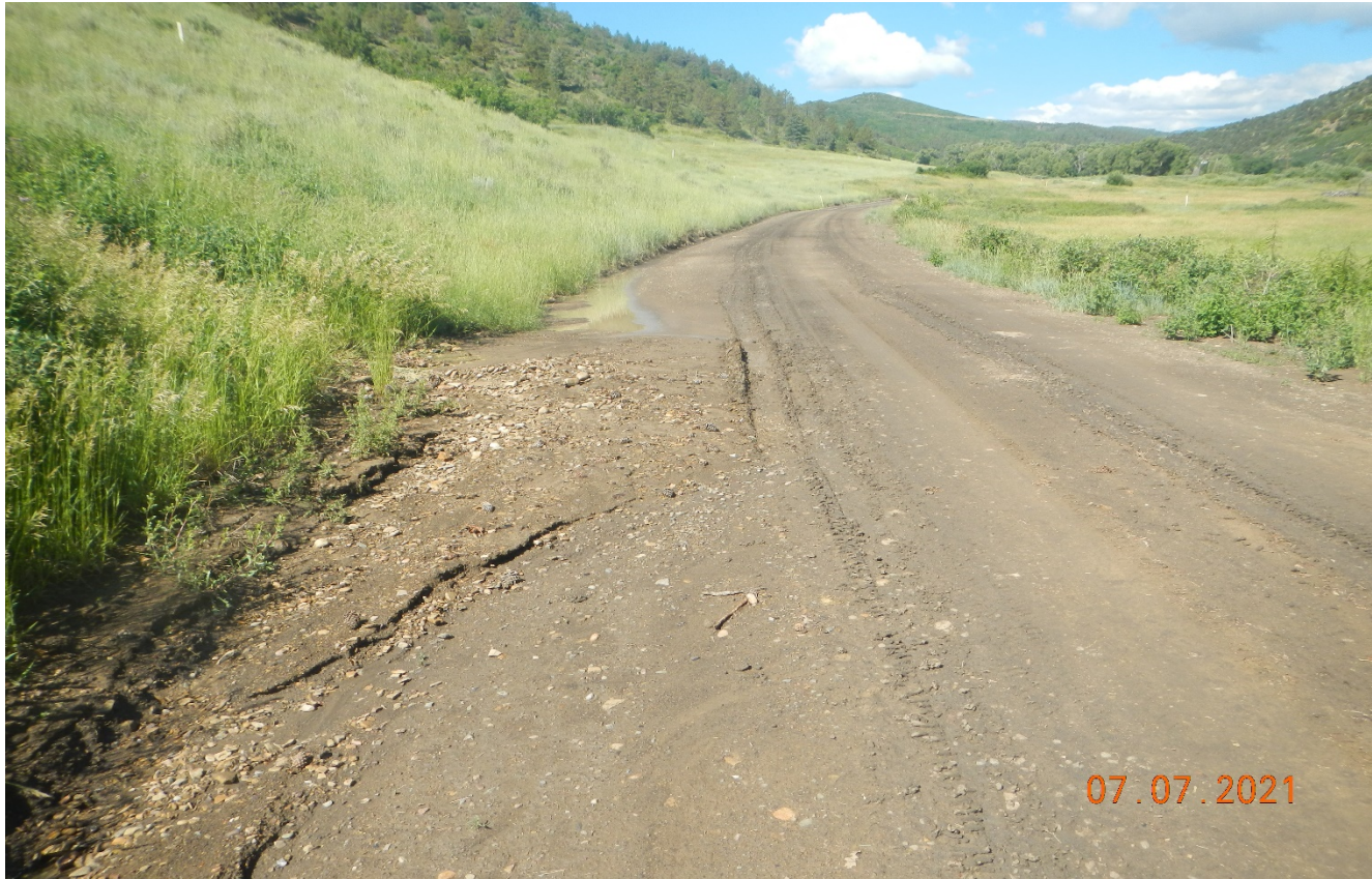
Photo 4. Sediment has washed into the road from recent rain event. The sediment needs to be removed to establish drainage toward the culvert.
