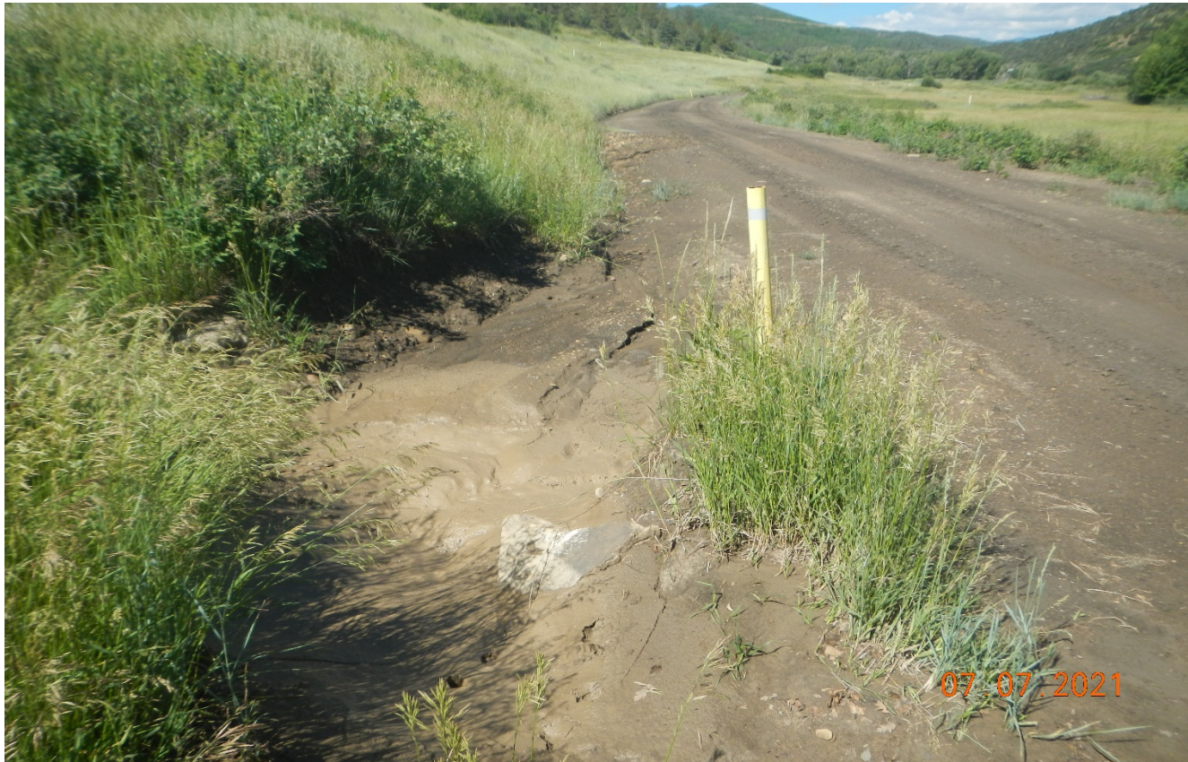
Photo 3. It appears recent rain events have deposited sediment into the culverts. Ongoing maintenance needs to be performed.
