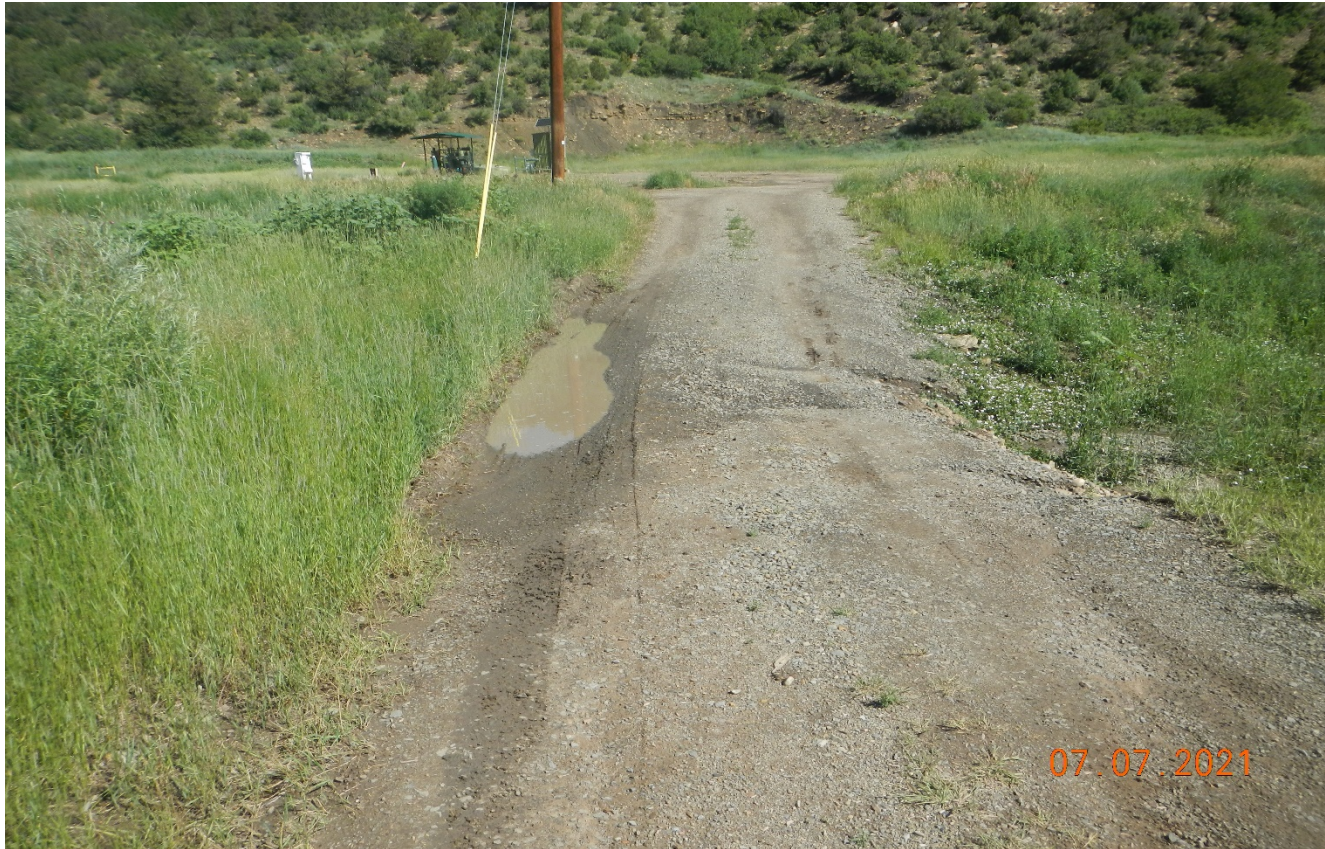
Photo 5. Facing northwest along the access road. This area of the road was not repaired. Stormwater is accumulating and has eroded across the road.
