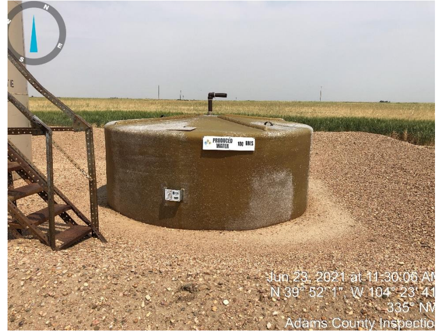
Photo #2 produced water tank.
