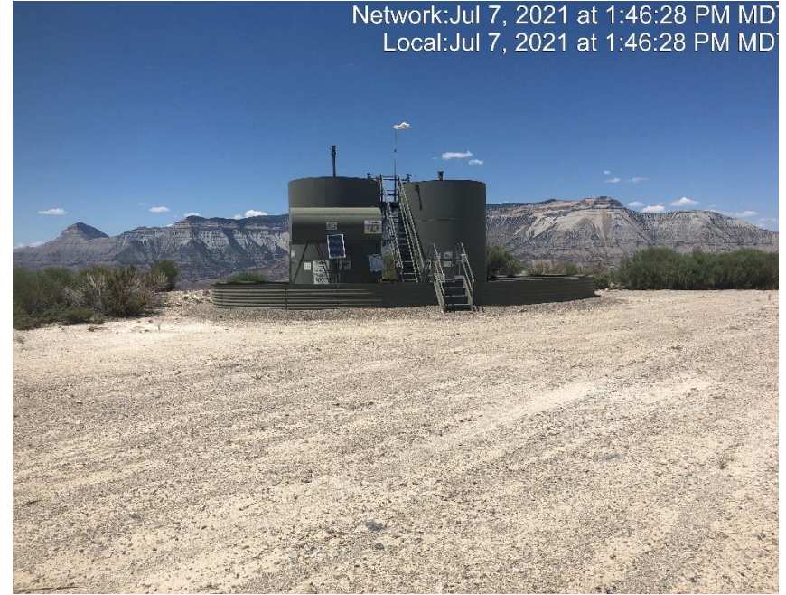
Photo #4344 No battery sign located at the tank battery.
