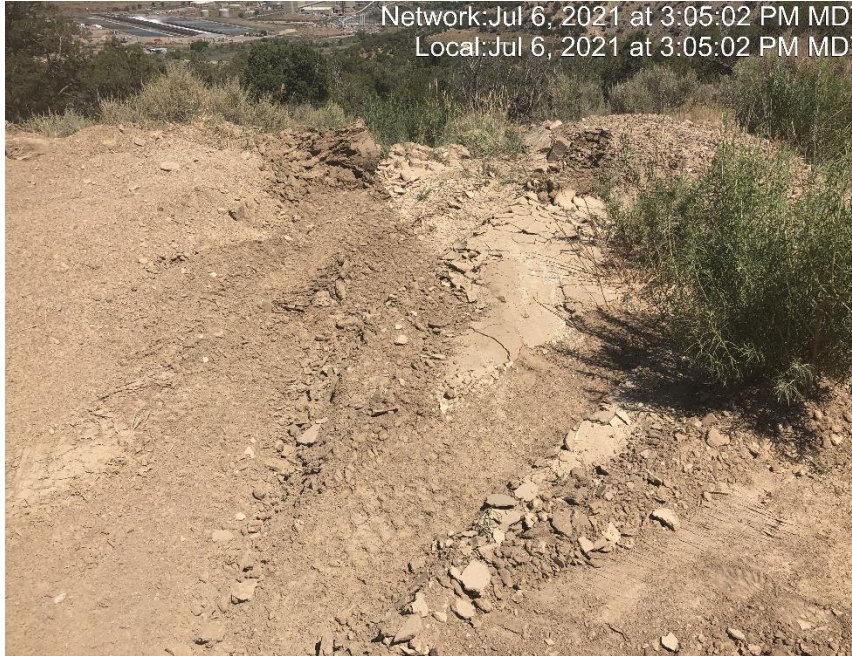
Photo #4329 Sediment trap insufficient.
