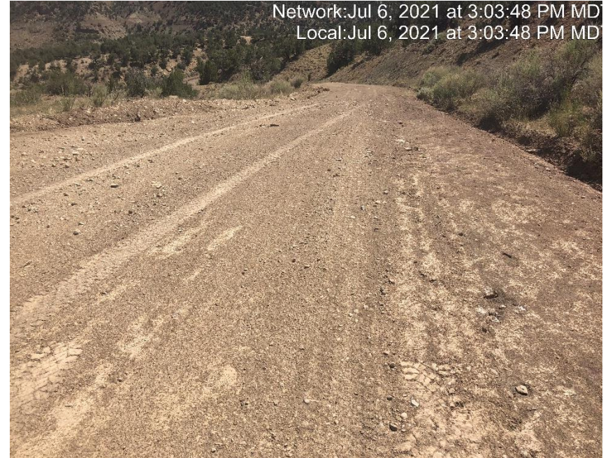
Photo #4327 Access road lacks stabilization.
