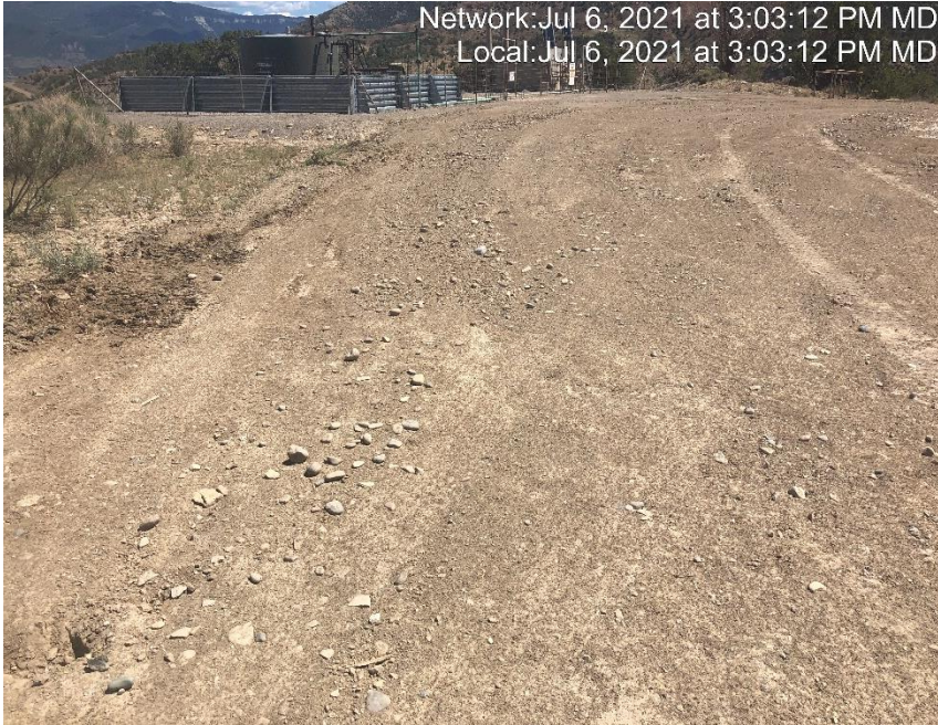
Photo #4326 Location lacks stabilization.
