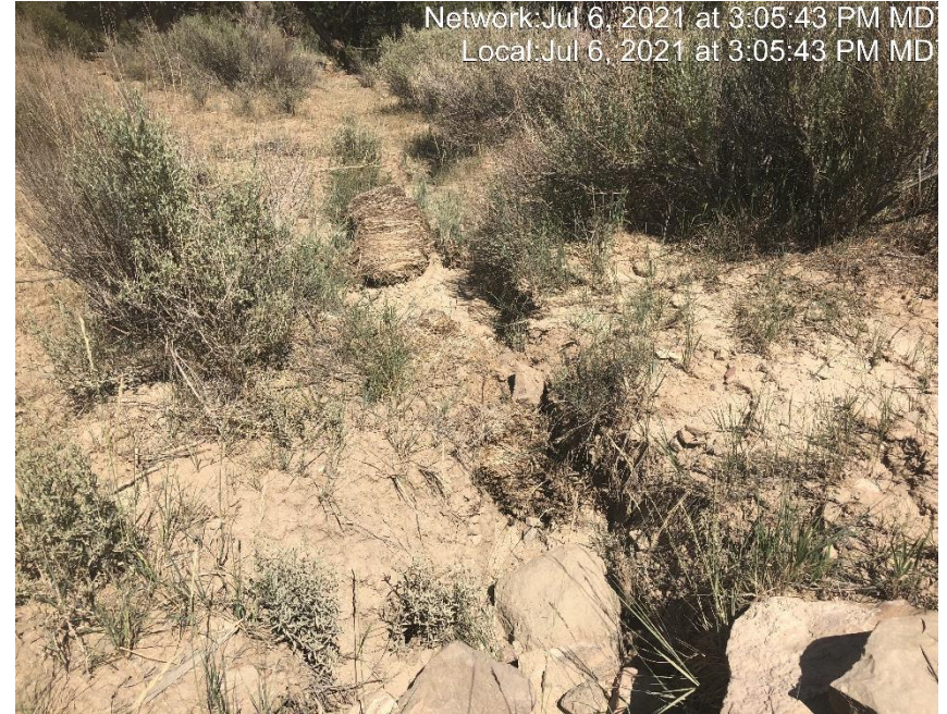
Photo #4331 Gully erosion occurring downstream of sediment trap.
