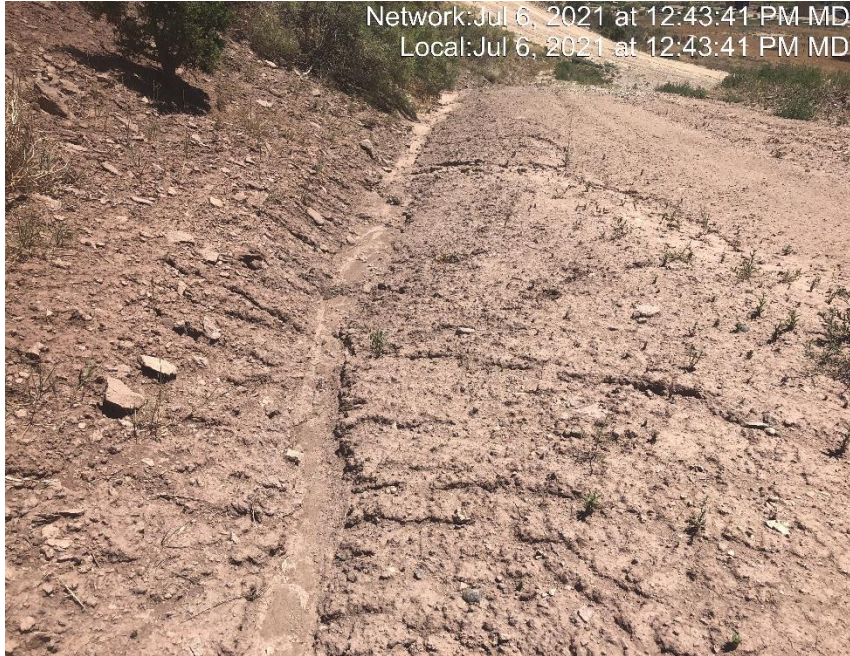
Photo #4310 Rill erosion occurring in access road ditch.
