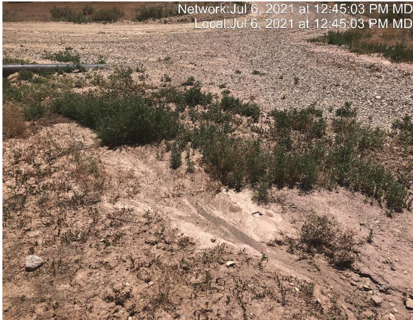
Photo #4312 Sediment accumulation at entrance to access road.
