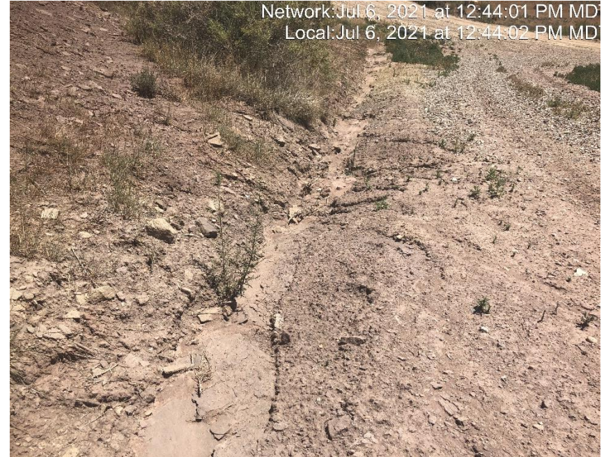
Photo #4311 Rill erosion occurring in access road ditch.
