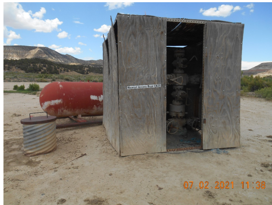
Injection Wellhead housing and propane tank.
