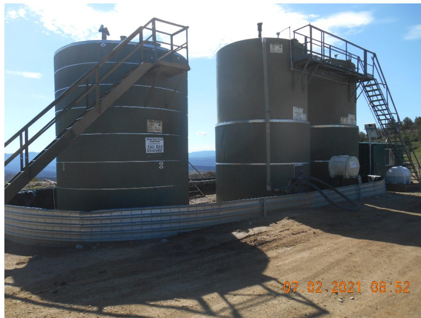
Tank battery and Secondary containment of chemicals
