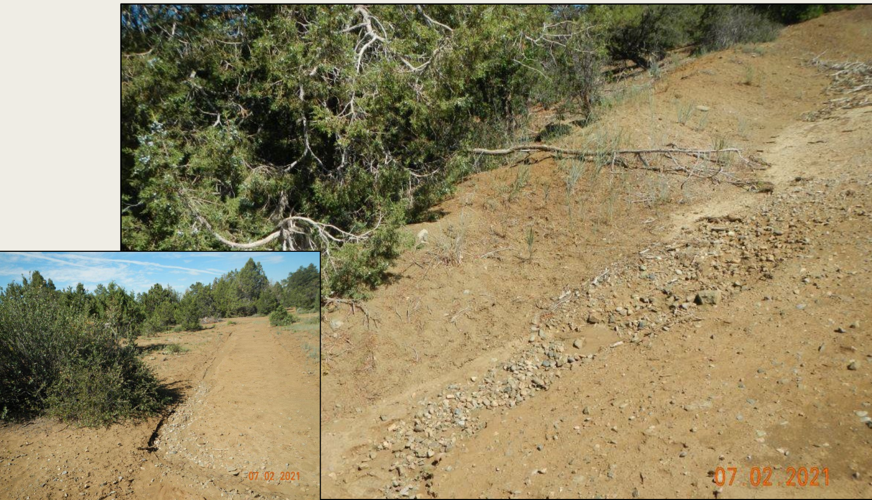
Photo 3. View of erosional channel forming (approximately 6 inches deep and 1.5 feet wide) and sediment deposition within the southwestern project area (facing upslope). Inset shows channel flowing off of the project area and downcutting.
