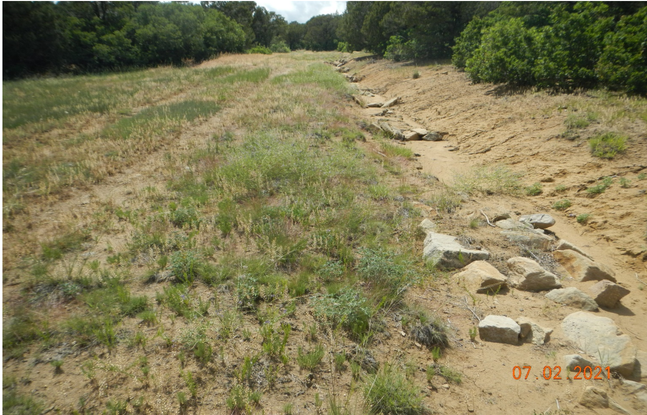
Photo 1. Facing southwest along the former access road. The road was not recontoured and reclaimed. There is erosion occurring along the road and the rock check dams are displaced.
