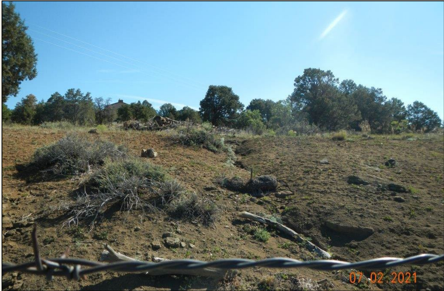
Photo 3. View of erosional channeling within the northeastern project area. Wattles are full of sediment and degrading. Green plastic debris present. These BMPs are not adequate and need to be installed using good engineering practices.
