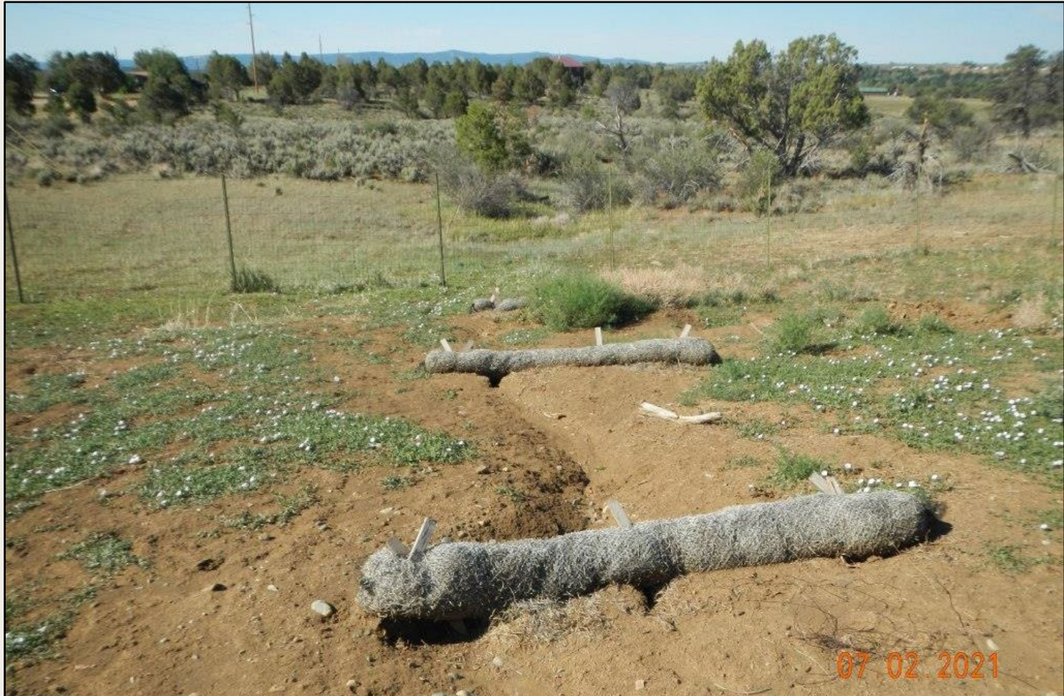
Photo 3. View of wattles and erosional channeling in the southern project area. Wattles are not an adequate BMP for this area. Little desirable vegetation present.
