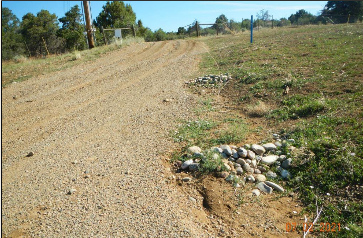
Photo 4. View of cobble BMPs along the access road, full of sediment and not functioning. These BMPs are not adequate and need to be installed using good engineering practices.
