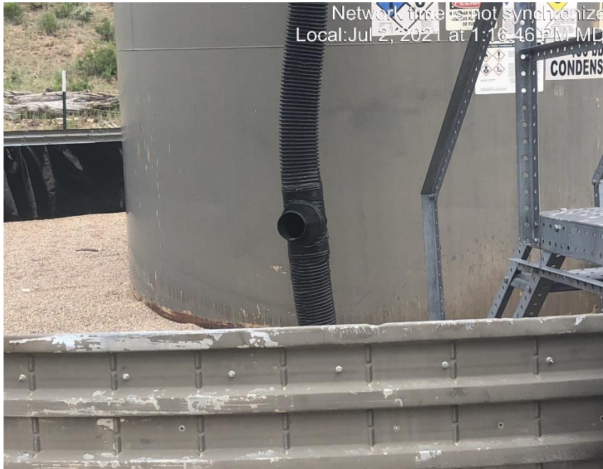
Photo #4300 Flow line heating insulation open ended and not capped.
