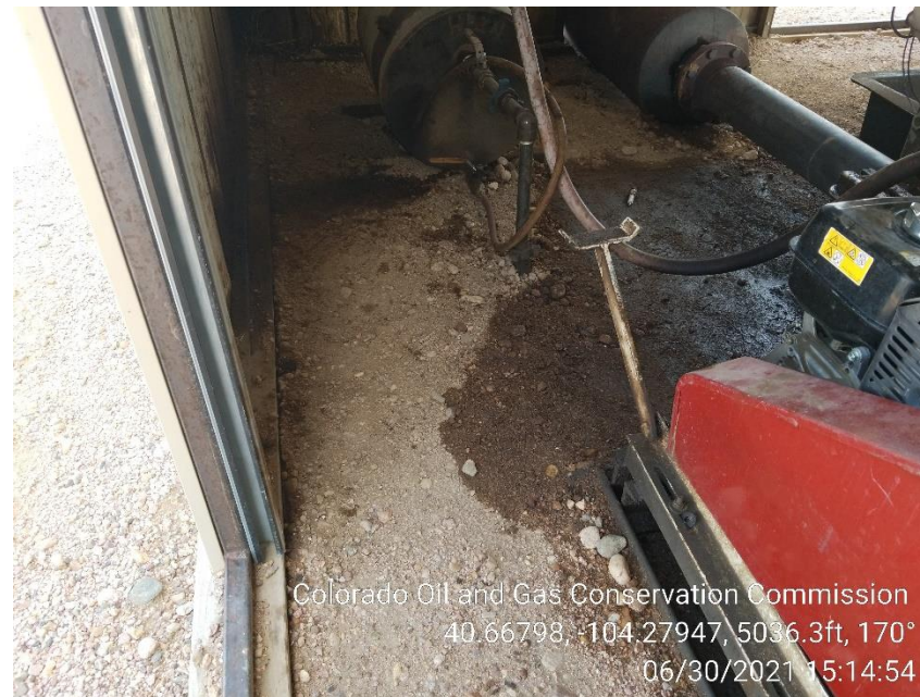
Photo 6 – Stained Soil at Gas Engine
