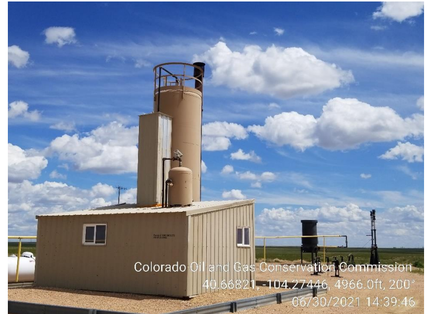
Photo 6 – Heater Treater, ECD and Flare
