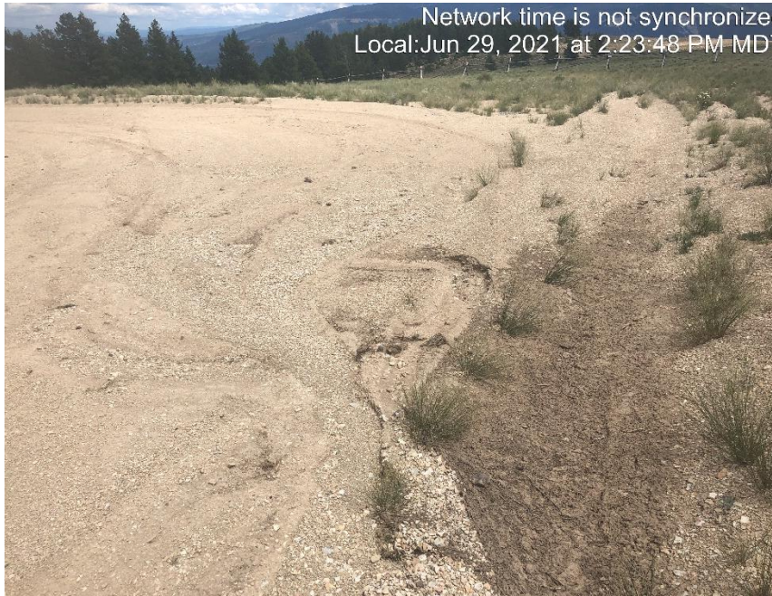
Photo #4233 Sediment accumulation at the corner of access road.
