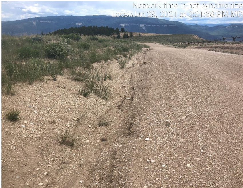
Photo #4229 Gully erosion occurring in access road ditch.
