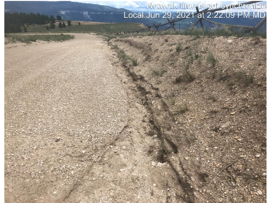
Photo #4230 Gully erosion occurring in access road ditch.
