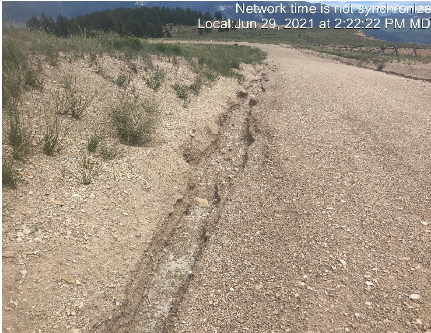
Photo #4231 No form of velocity check.
