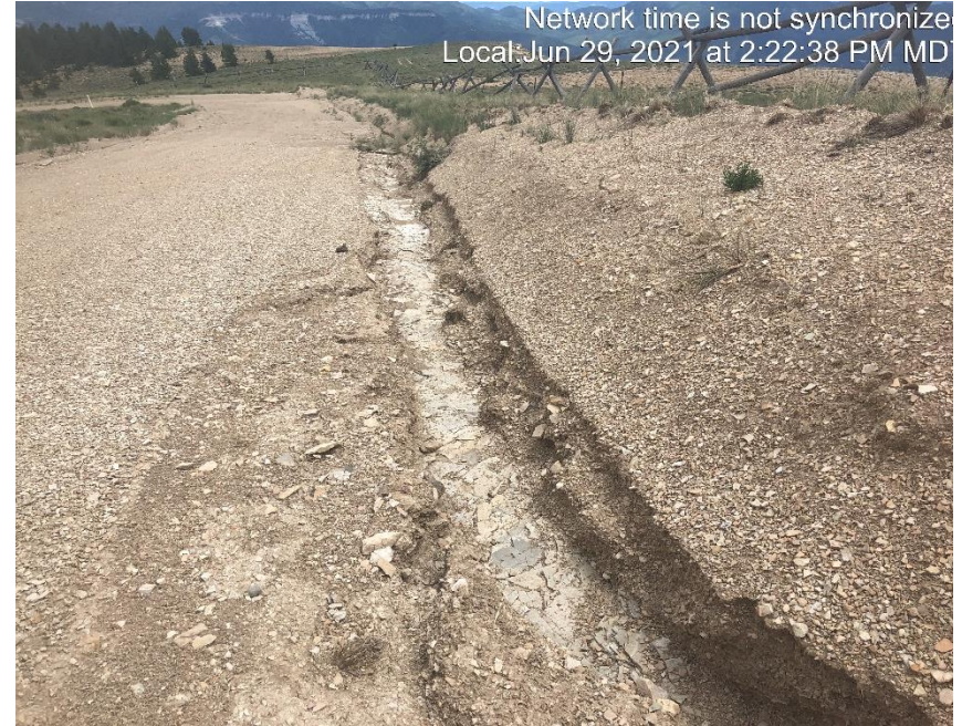
Photo #4232 No form of velocity check.
