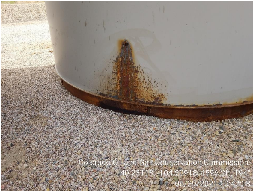
Photo 7 – Leak on Tank; addressed
