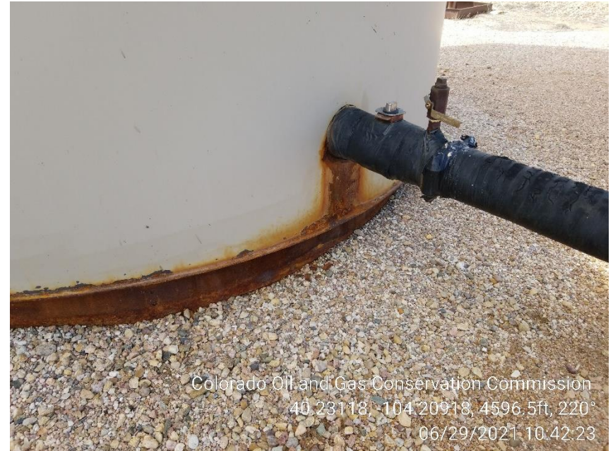
Photo 6 – Loadline leak; addressed
