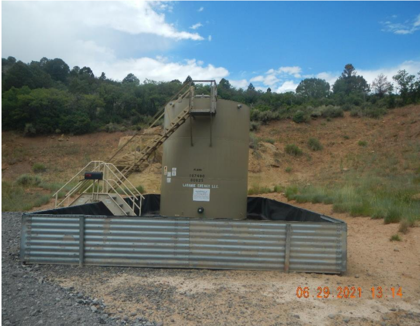
No battery sign at tank battery.
