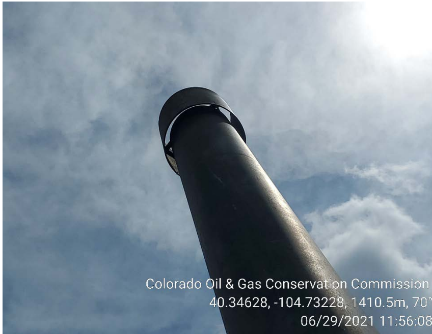
Separator burner stack
