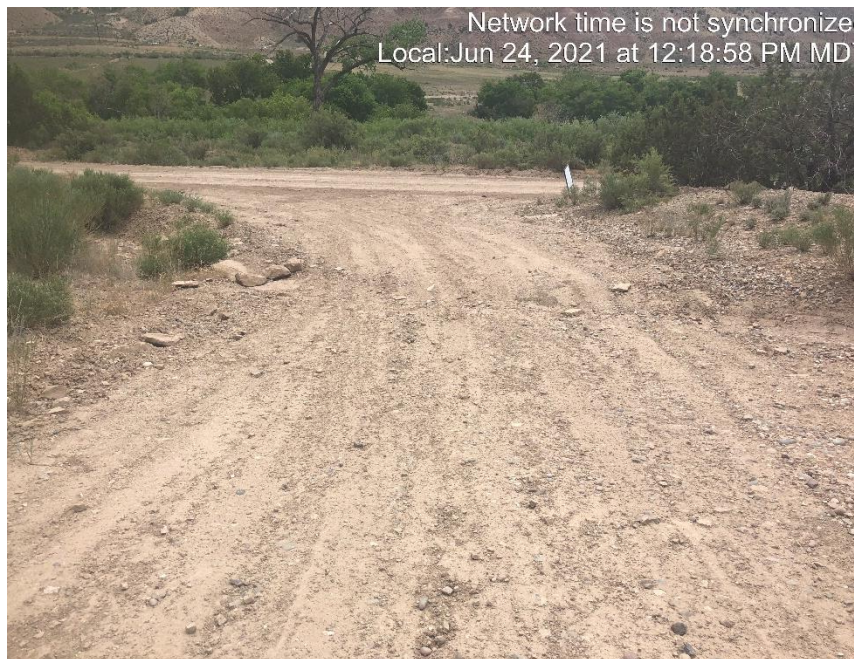
Photo #4165 No form of tracking BMP located at the entrance to location.
