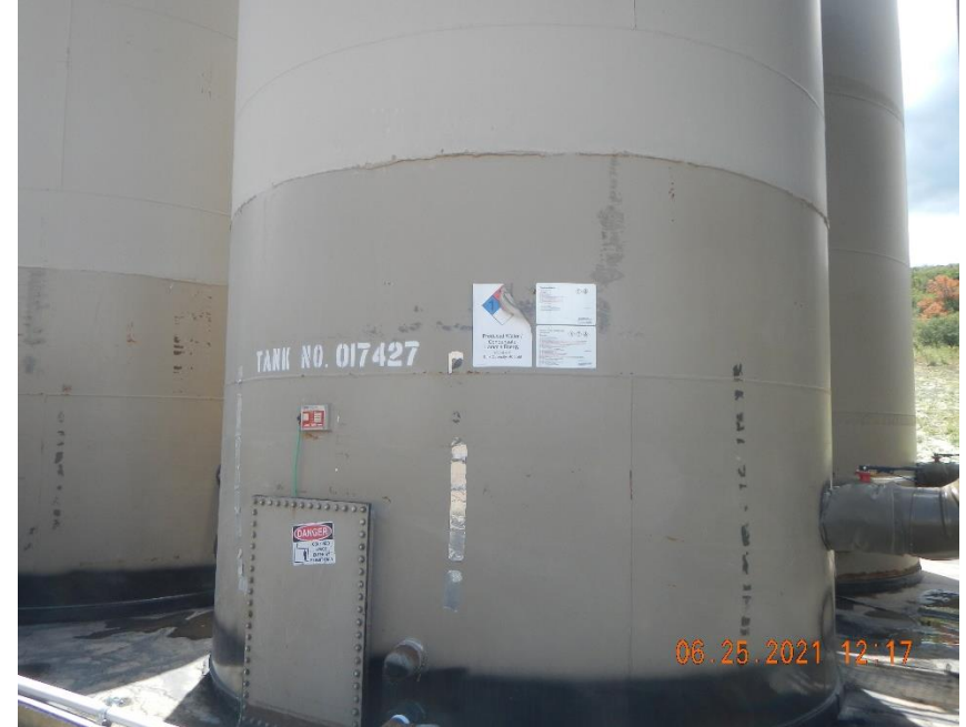
Label is not fully adhering to tank.
