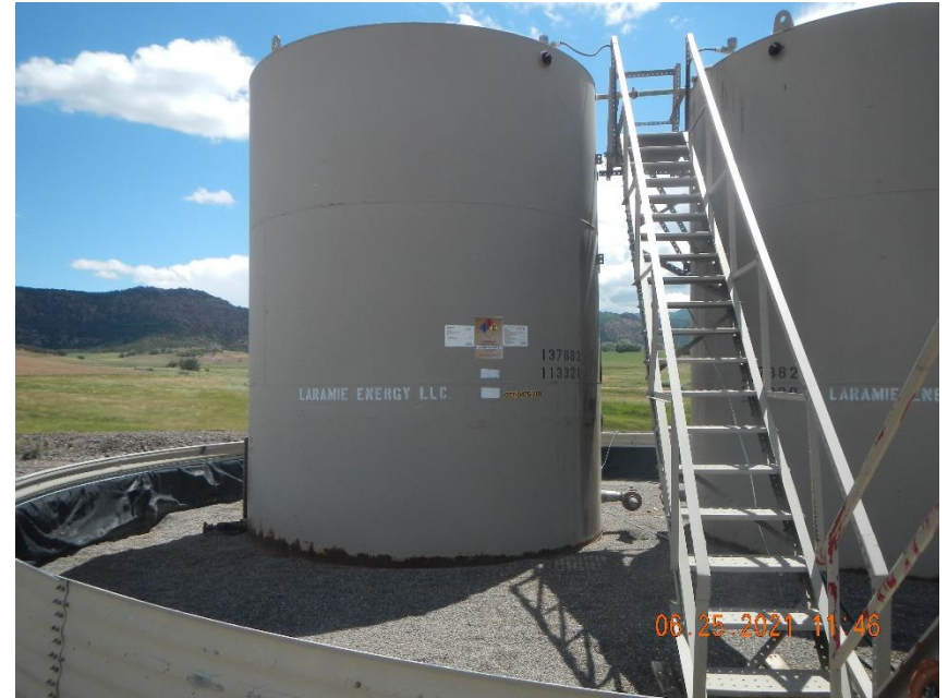
Tank label is discolored and illegible from a distance. (100')
