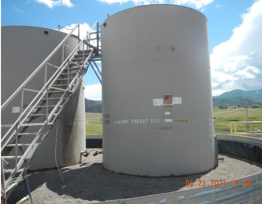
Tank label is discolored and illegible from a distance. (100')
