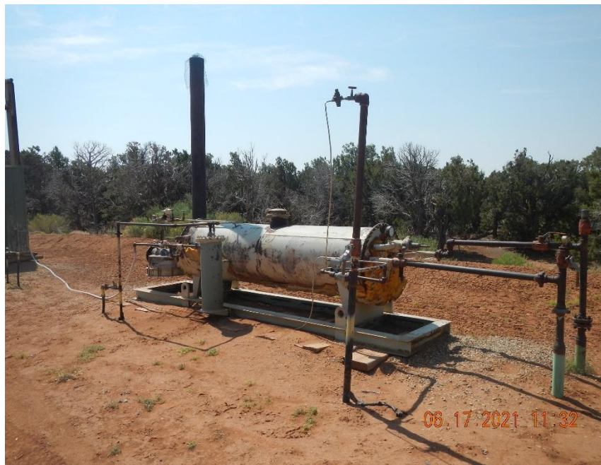
Horizontal heated treater in SW corner of location.
