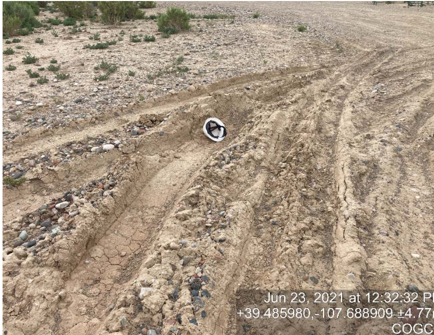
Lack of stabilization/compaction
