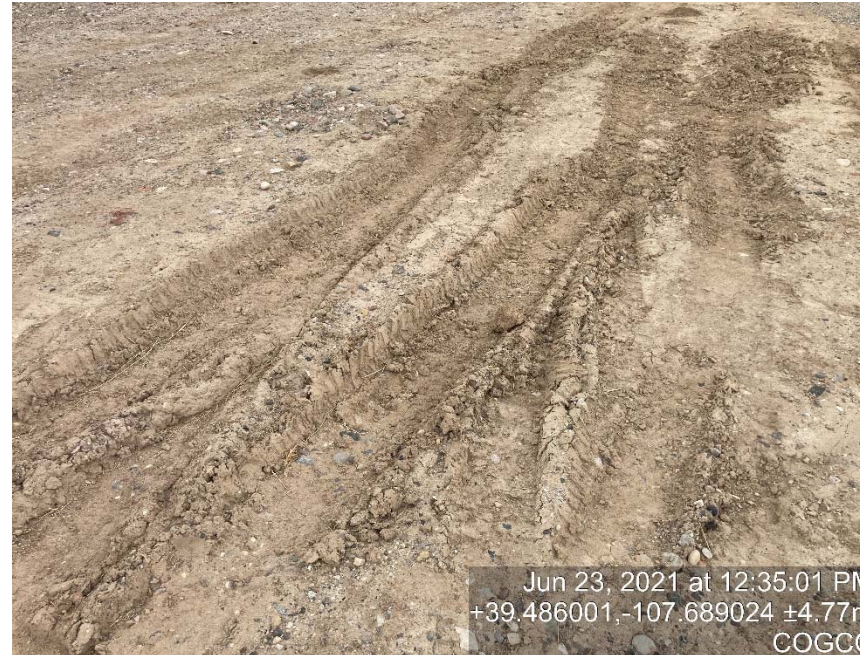
Lack of stabilization/compaction
