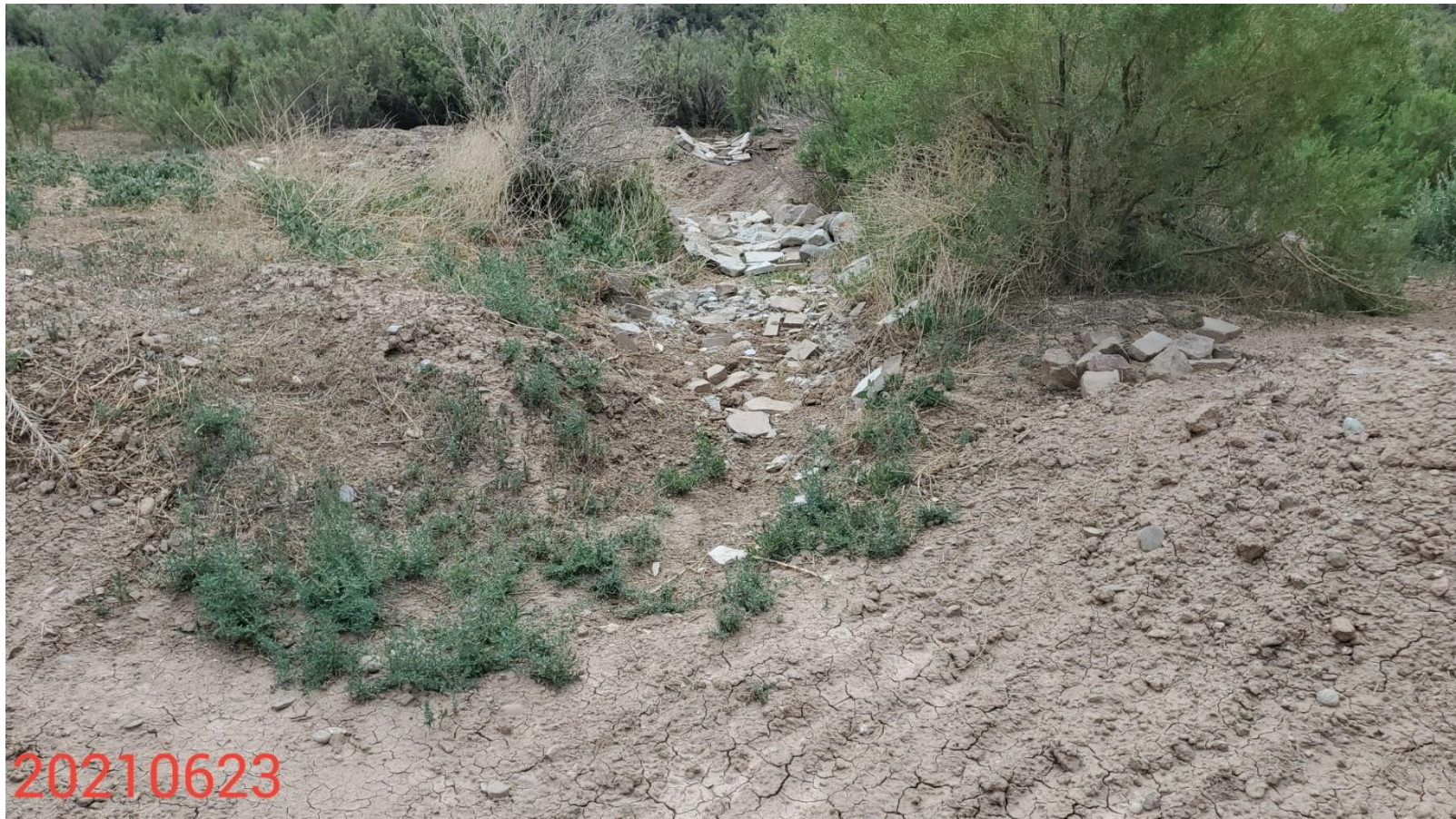
Photo 9: Photo taken from the southeast end of the Location, facing east. Photo shows sediment trap.
