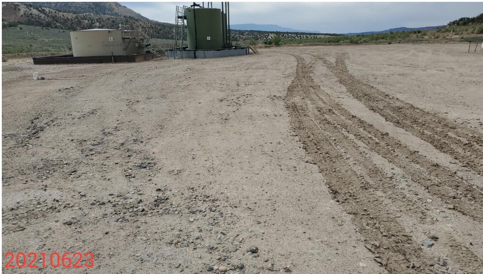
Photo 1: Photo taken from north end of the Location, facing south. Photos 1-3 provide and overview of the Location from south, southwest to west. Photo shows control measure to stabilize/protect the production areas, or to prevent off-site sediment transport and tacking remain missing or insufficient
