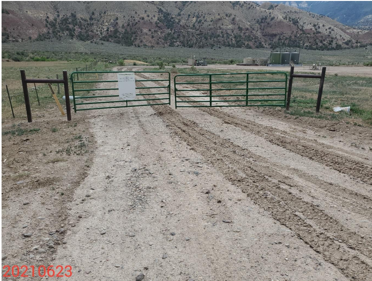
Photo 4: Photo taken from the Location entrance, facing east. Photo shows tracking and off-site sediment concerns remain evident; control measure to stabilize/protect the production areas and access road, or to prevent off-site sediment transport and tacking remain missing or insufficient
