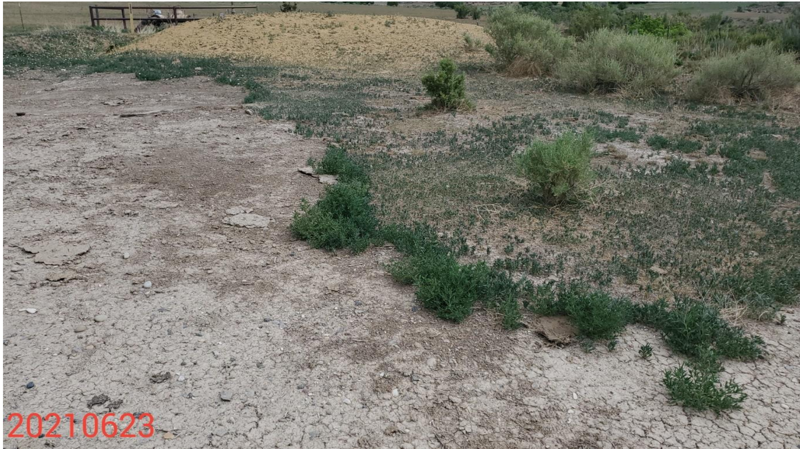
Photo 12: Photo taken from the northwest corner of the Location, facing north. Photo shows hydromulch has been applied to the soil stockpile. Photo also shows undesirable weedy plant establishment remains evident
