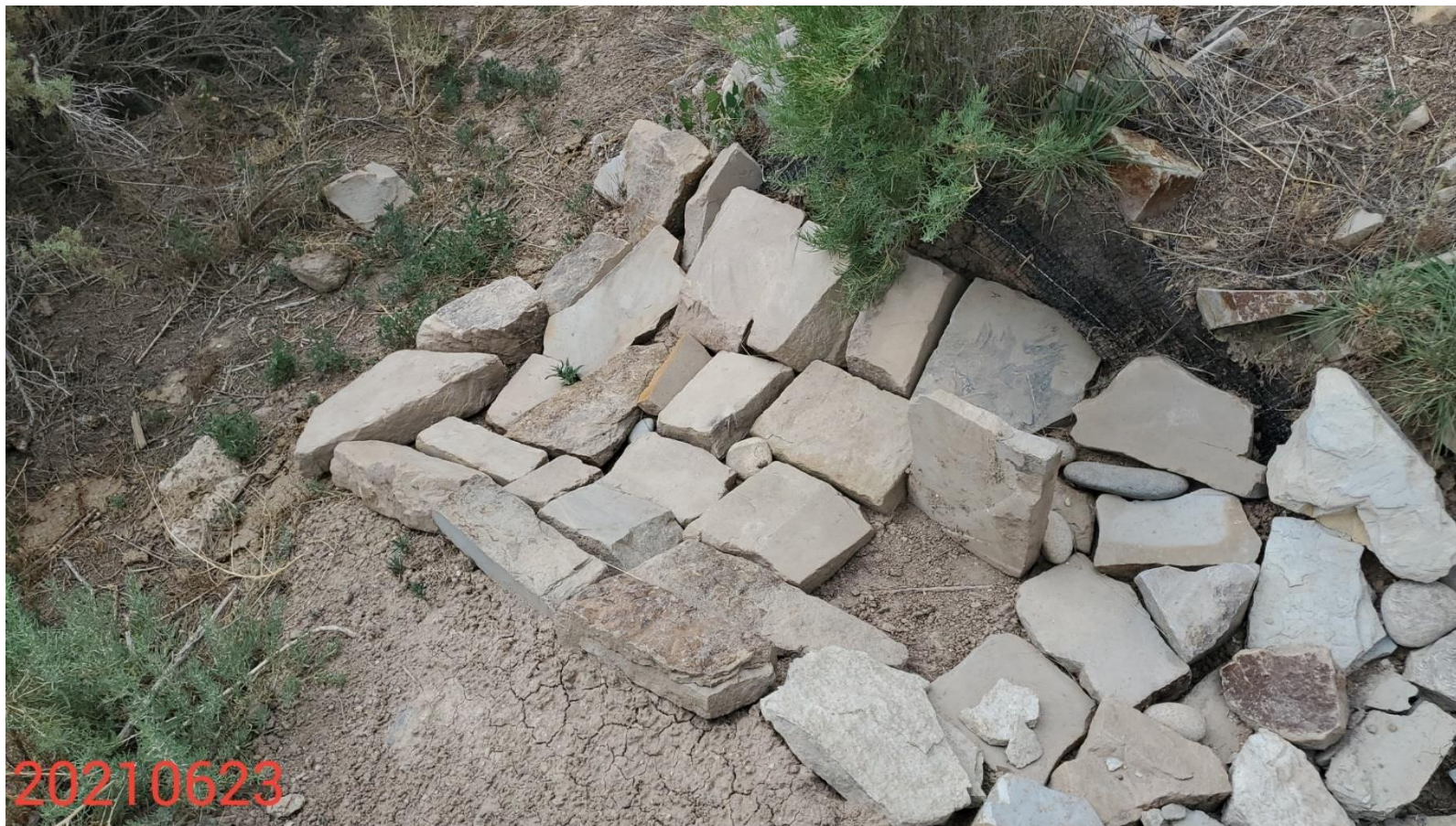
Photo 10: Continued from photo 9. Phot shows sediment trap has not been constructed with geotextile lining in accordance with good engineering practices
