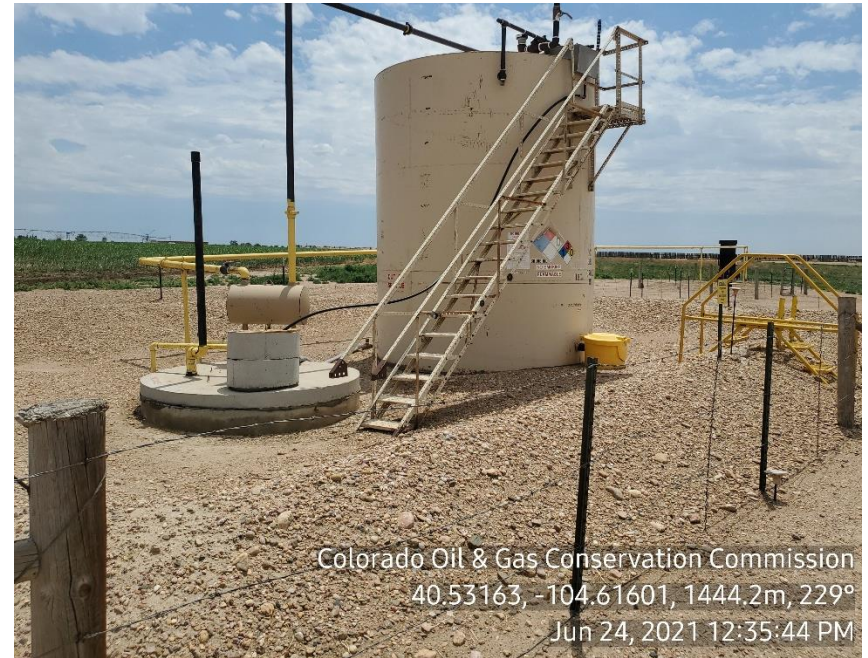
Photo 4: Tank Battery
